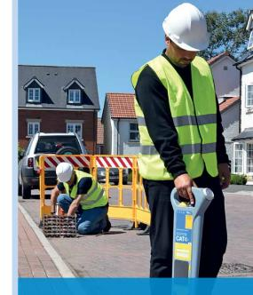
Trace non-metallic utilities Accurately trace non-metallic pipes or telecom ducts using sondes.
